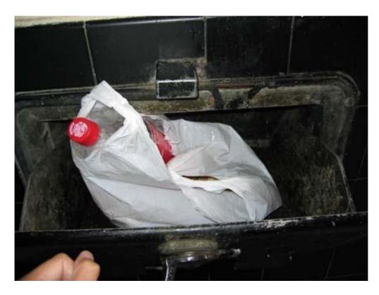
At least one hopper head within the block is blocked with rubbish. There may also be evidence of rotting food and/or maggots within the hopper head.
