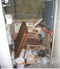
The intake cupboards are full of toys and building materials or full of rubbish and litter obstructing switches or meters etc. The condition would constitute a fire hazard and encourage vermin.
